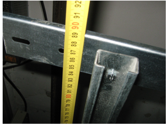
Barrier in Higher Position
